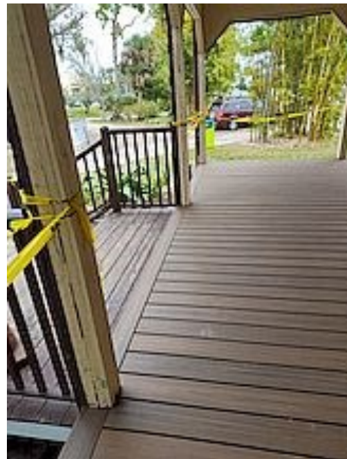
Entry steps and porch decking
