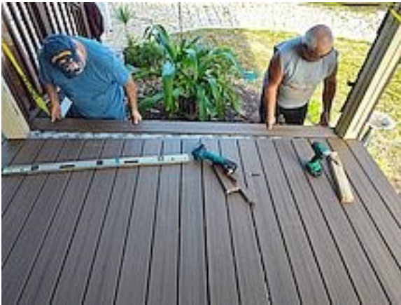
Ken Carteaux and Dave Arruda laying the porch edging
