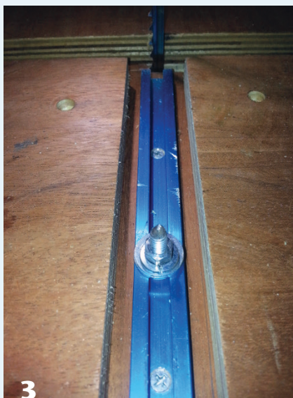
3 Add a second layer of plywood, leaving space around the blade and pivot track.
